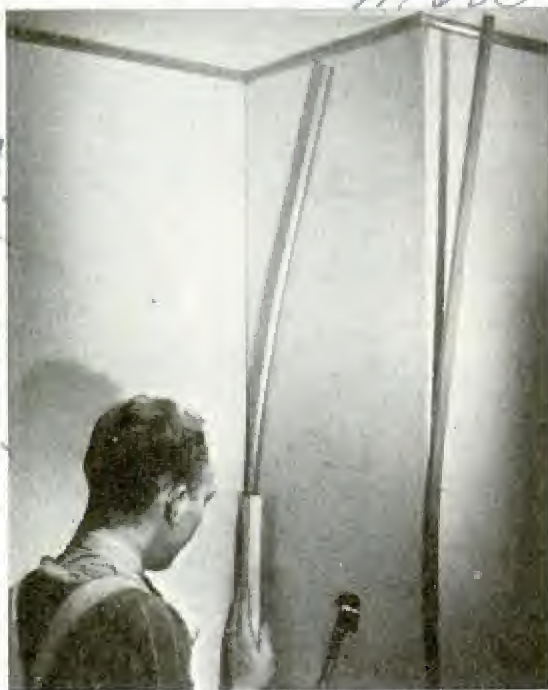
Plastic molding holds firmly when pounded into seam
